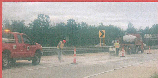
US-10 Concrete Work
