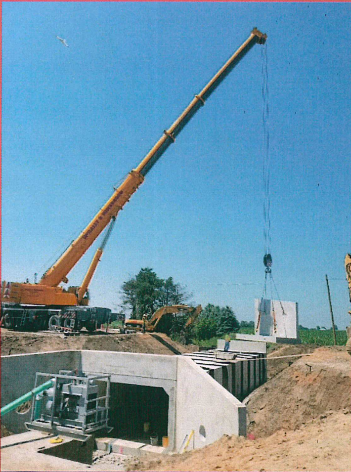
Mackinaw Road Reconstruction
