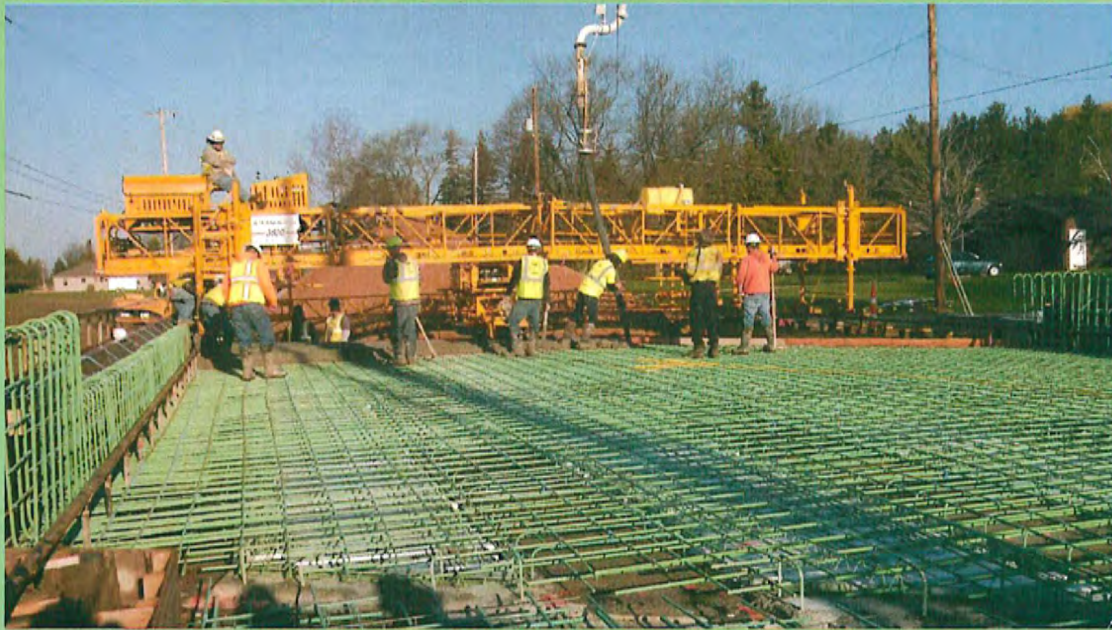
Midland Road Bridge Construction
