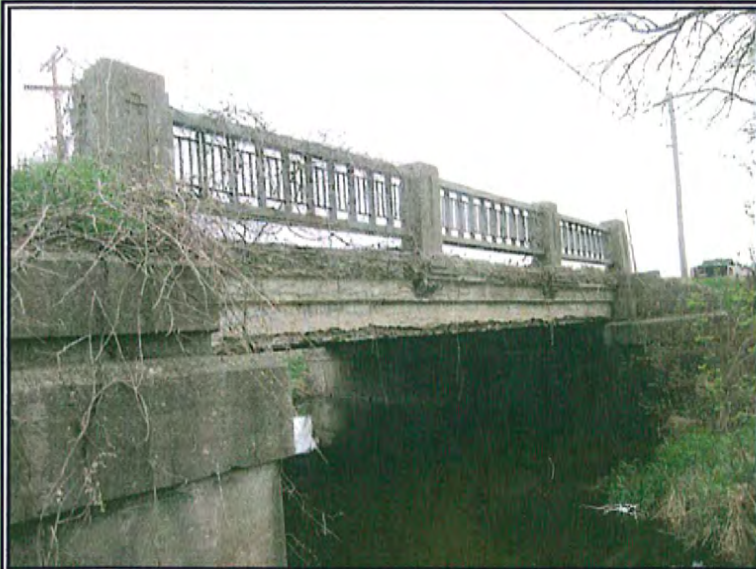
Midland Road Bridge Before
